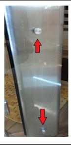
Align the holes in the back of the heater with the holes on the door.
