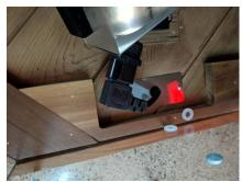
Now working backwards, plug your new heater into the floor cord and tuck the connection back into the opening on the bottom of the heater.
